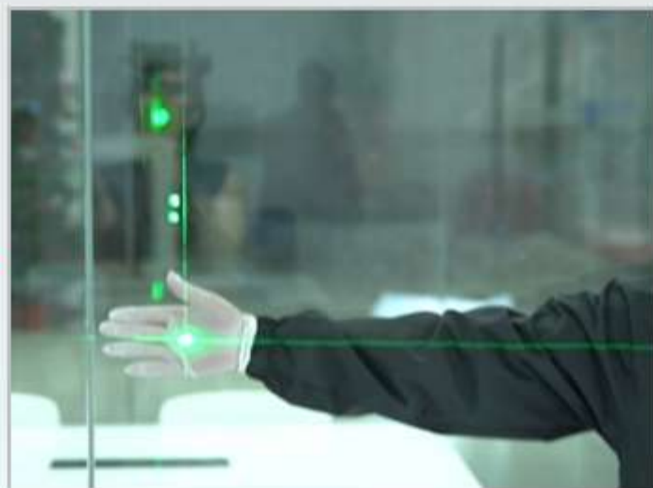
Step 2. Make a horizontal line on the installation position.
