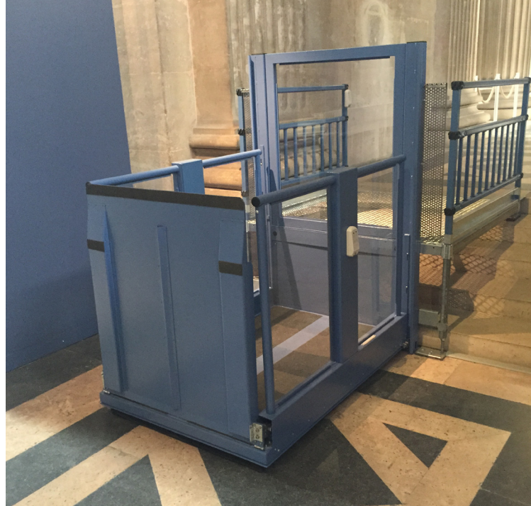
Access ramp instead of door on the platform
